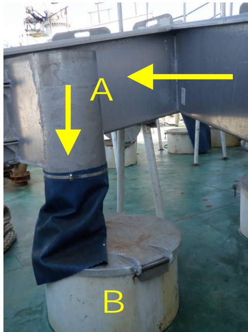
Figure 7. Detail of channelization (A) into the holding tank (B)
